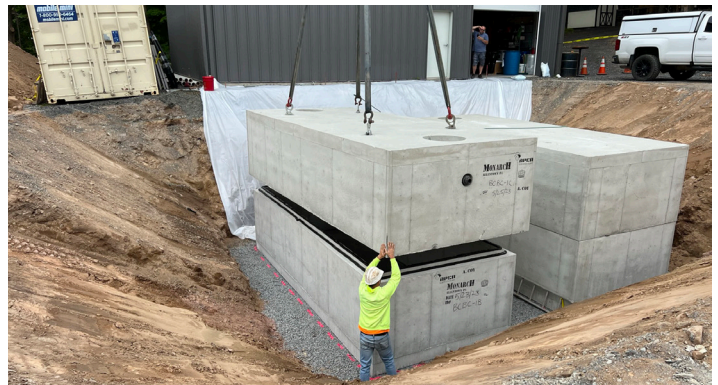
(Top) Aeration and sludge settling tank within the treatment process (Bottom) Installation of the underground equalization tank during construction
