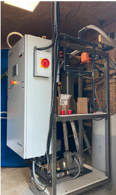
Compact & Efficient MBR System - On-site treatment removes 99% of BOD for safe discharge.
