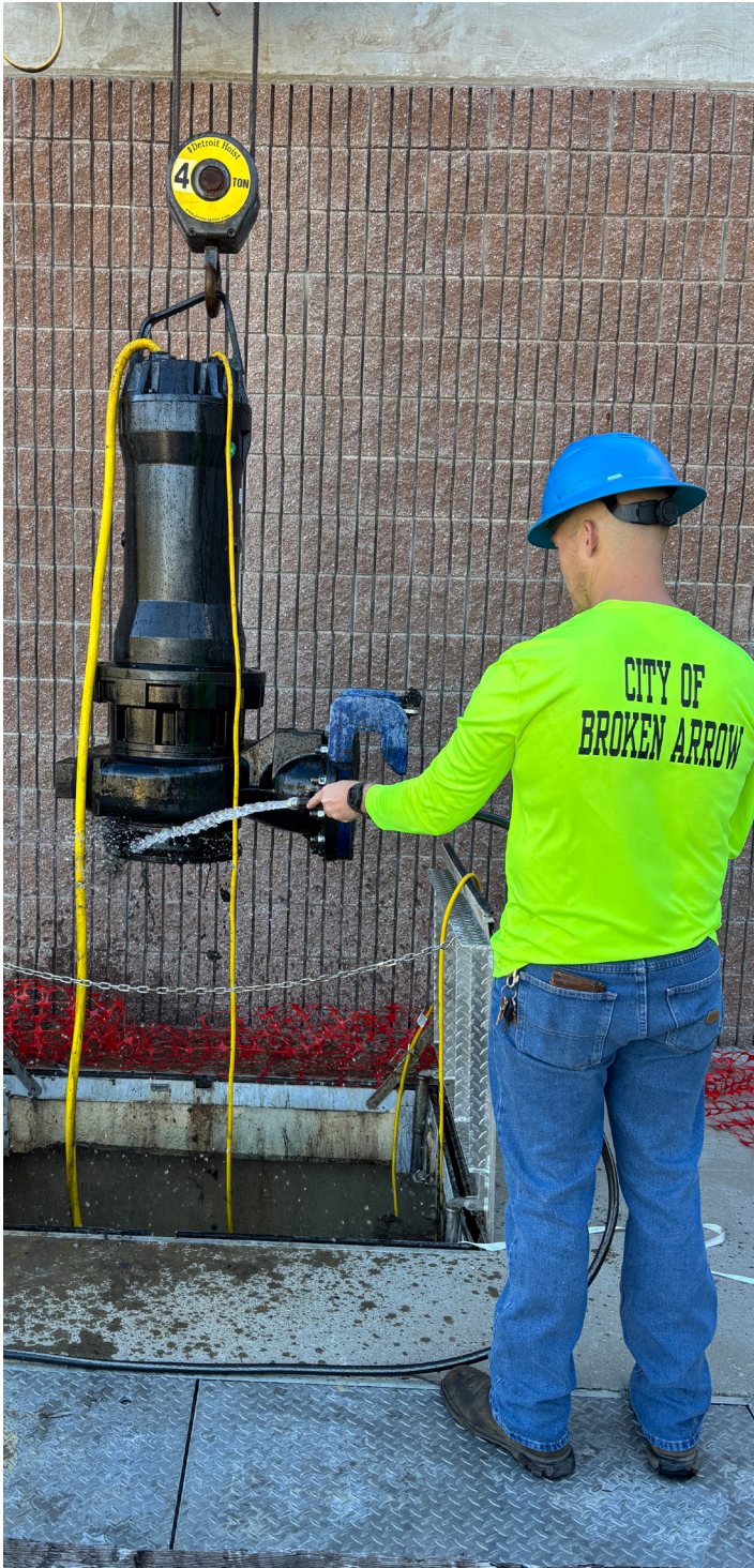
Lift station operator guiding installation of the AVANT MQB submersible pump to improve performance in demanding wastewater conditions.
