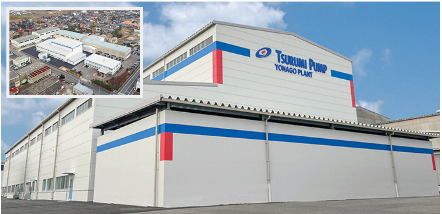
Tsurumi Yonago Plant, located in Tottori Prefecture, Japan, is equipped for advanced manufacturing and performance validation
