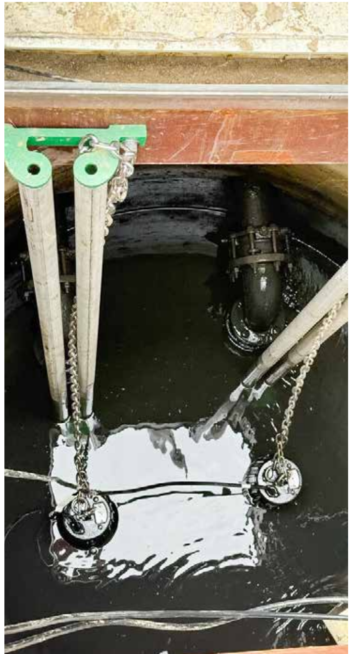
Retrofit success: Tsurumi C Series Cutter Pump™ installed in an existing wastewater chamber for seamless integration and solids-handling.
