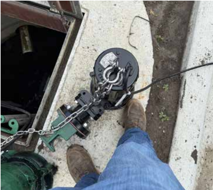
Pre-installation view of Tsurumi Cutter Pump™ for truck stop system upgrade.
