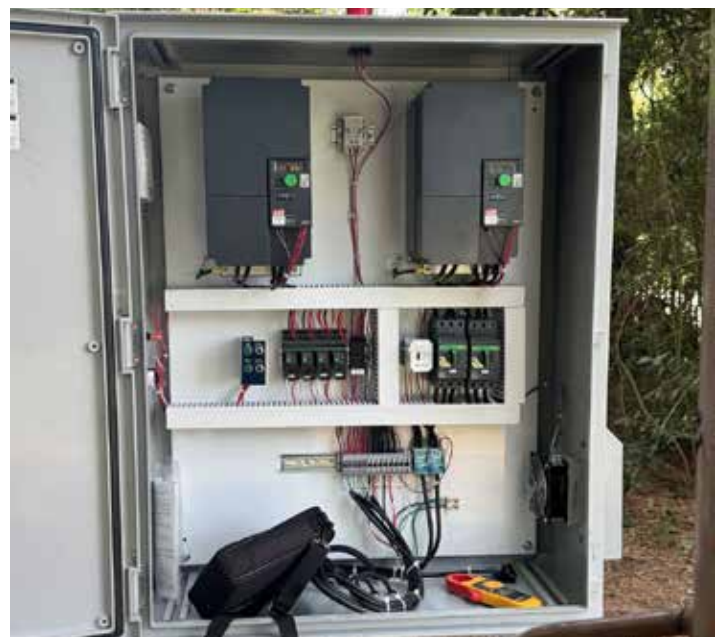
Upgraded with a Tsurumi inverter panel for smarter protection and control.
