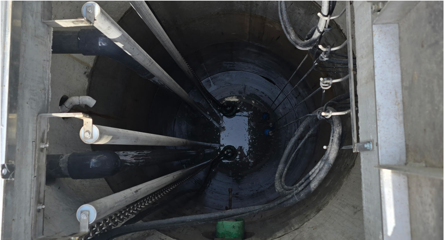
Tsurumi MYCZ pumps restore reliable, clog-free operation at a hospital's wastewater lift station in Florida.
