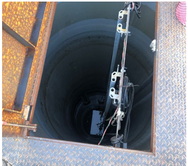
MBR system with Tsurumi VANCS™ pumps, BER aerators, MG grinder pumps, and guiderails.
